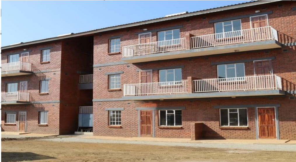
Dzivarasekwa Civil Servants Flat
