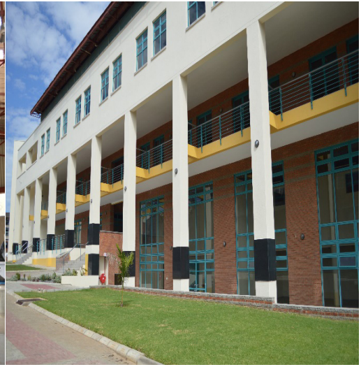
NUST Technovation Centre Block B
