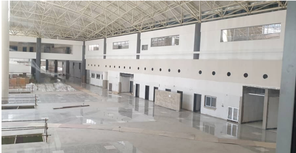
Inside of the Terminal Building
