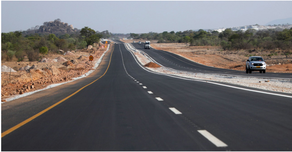
Harare- Masvingo- Beitbridge Road
