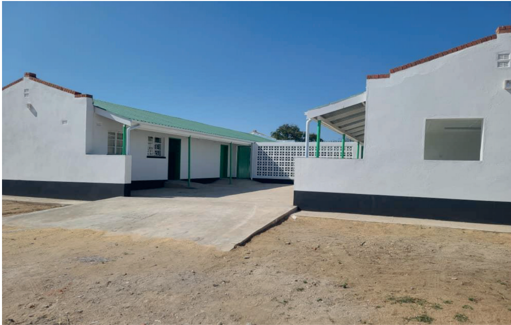
Umlugulu Clinic, Matobo RDC, Matabeleland South
