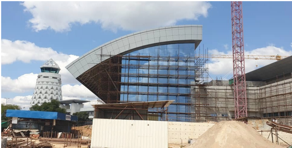
Outside of the Terminal Building
