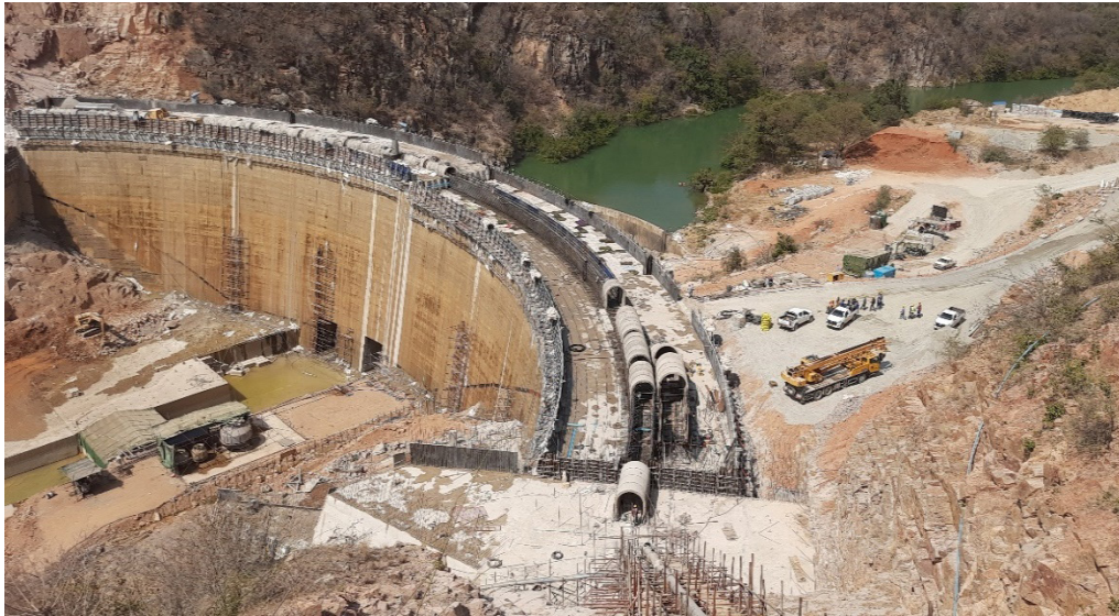
Gwayi Shangani Dam
