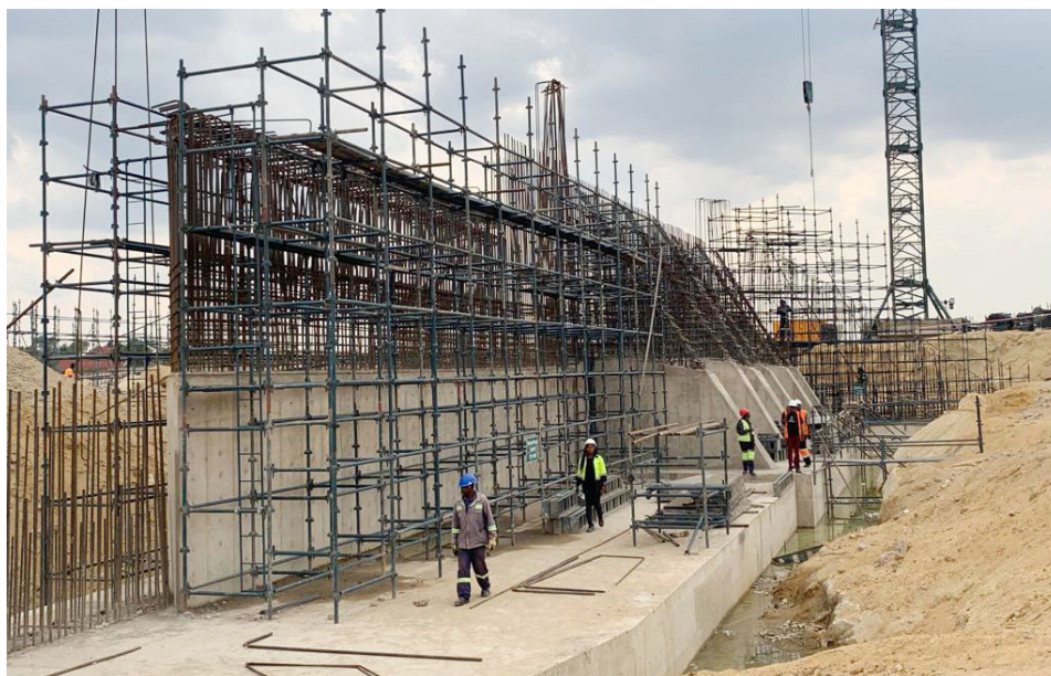
Mbudzi Interchange Construction
