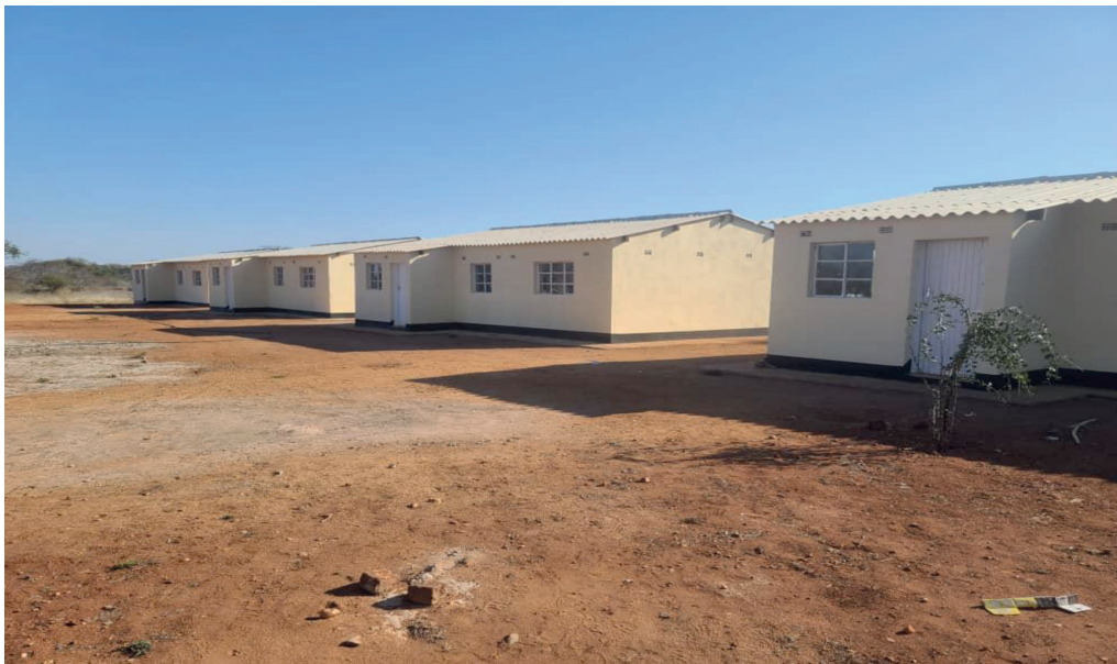
Mandihongola RHC Staff Houses, Gwanda RDC, Matabeleland South
