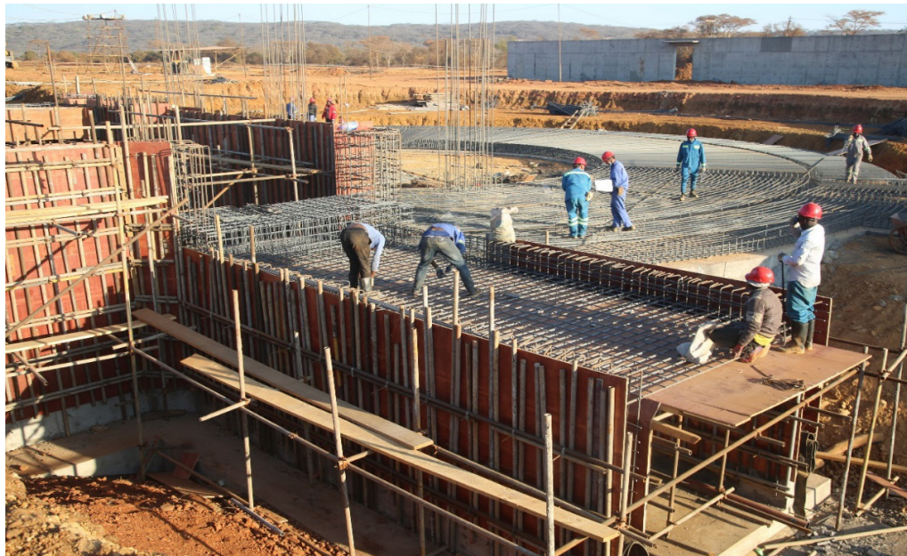
Construction at Manhize
